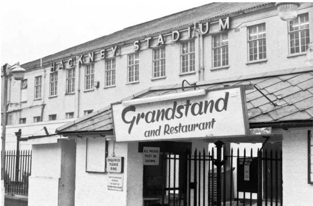
View of the Hackney Stadium entrance.
