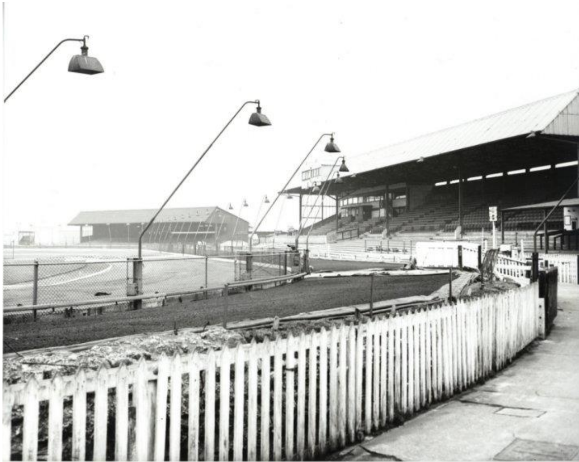
New Cross Stadium (Copyright – GRA)
